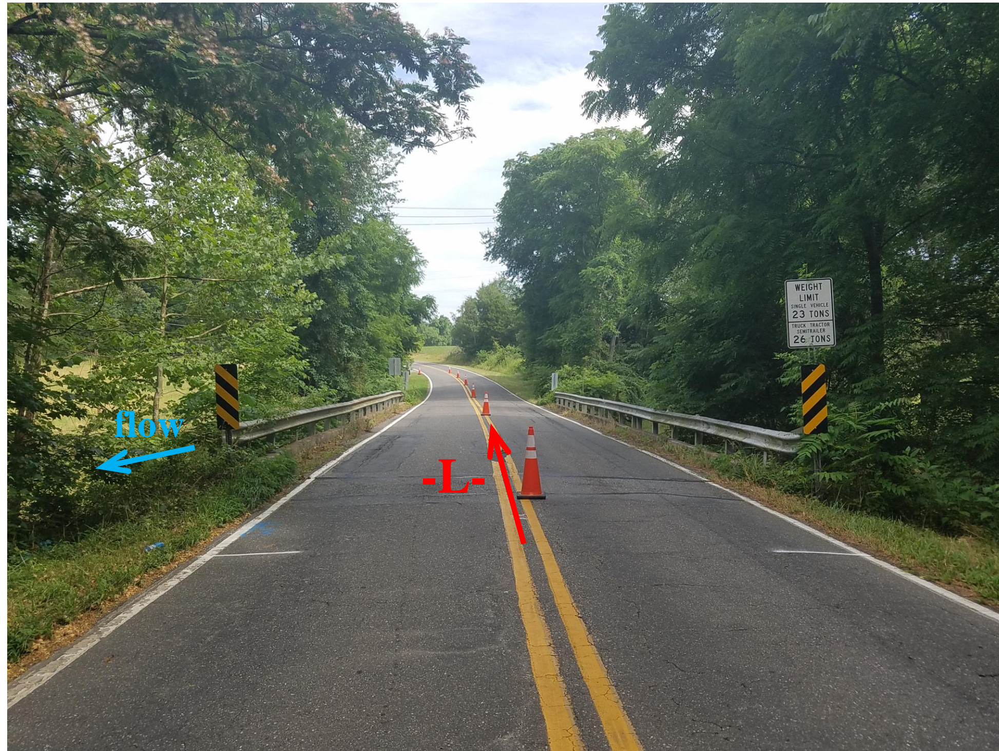
Looking North towards End Bent 2
